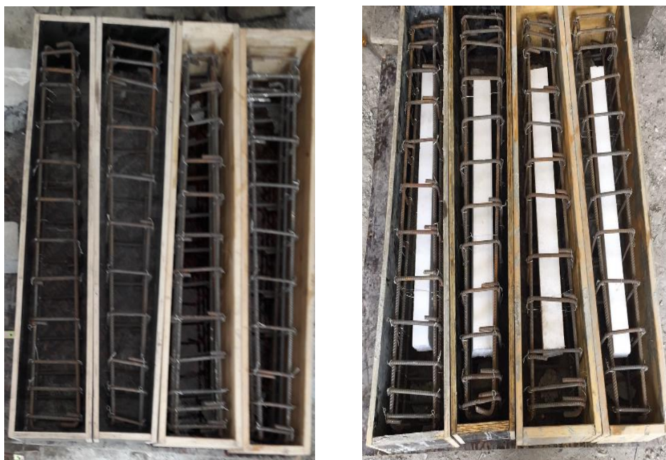
Fig.1 Moulds Fabrication and Reinforcement Layout .
