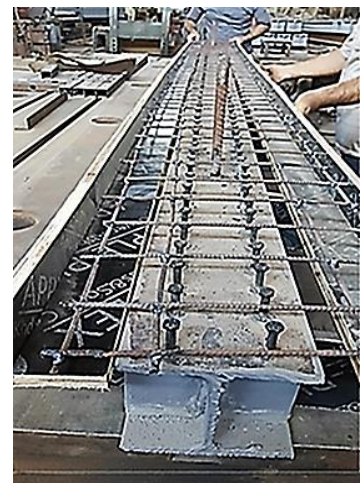
Fig. 6 Photo of the Slab Mould
