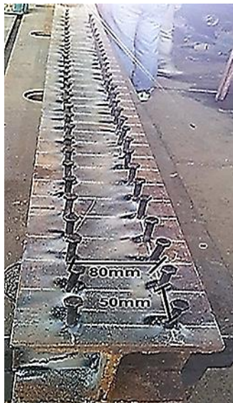
Fig. 2 Shear Connectors
