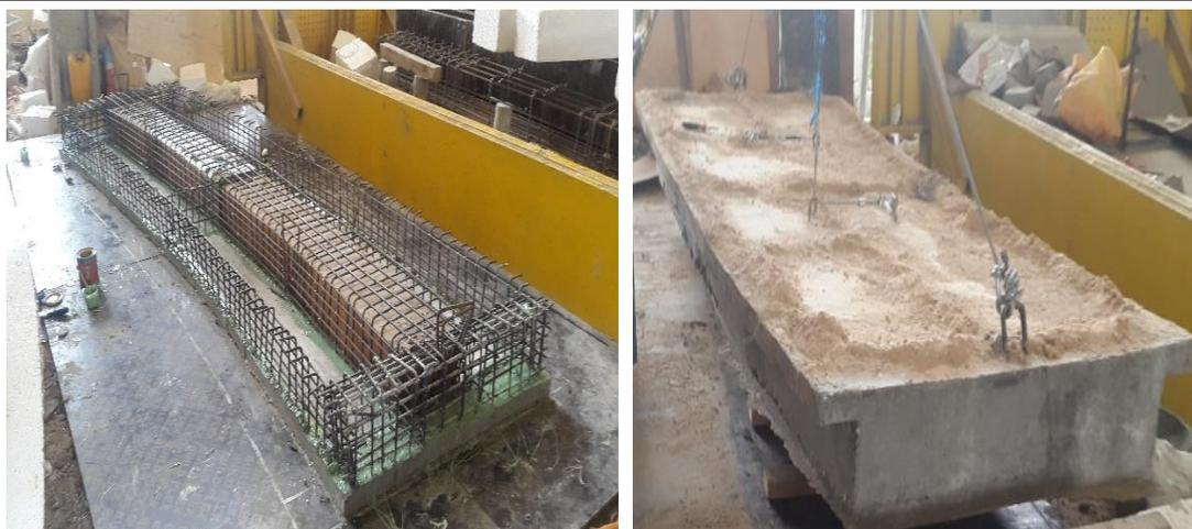
**Fig. 2 First stage of BGC R12.5 construction**
