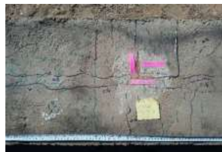
(c) Lateral crushing of concrete deck
