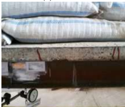
(b) Flexural cracks side view
