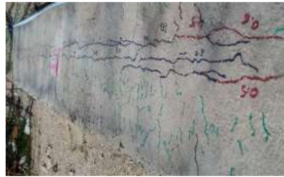
(c) Longitudinal concrete deck cracks
