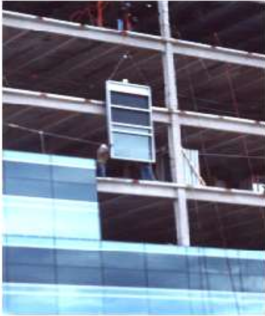
Fig. 4. Example of unitized system curtain walls
