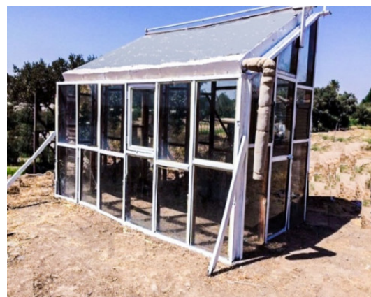
Figure 2: Show the wooden truss of the greenhouse.
