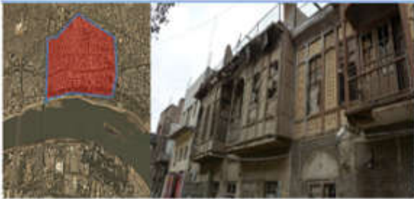
Figure 2: Desolated situation in residential neighborhoods heritage of Albatavin, [7]
