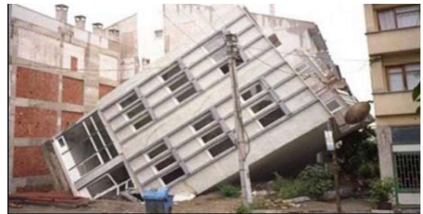
Figure 5: an example of Liquefaction Damage [6]
