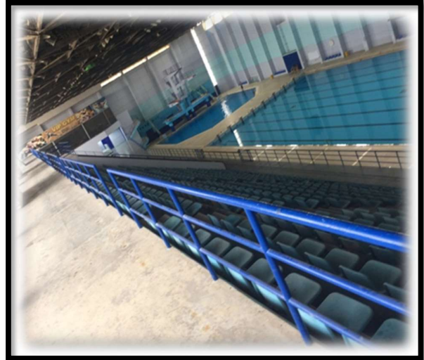
Figure 4: Building with indoor swimming pool
