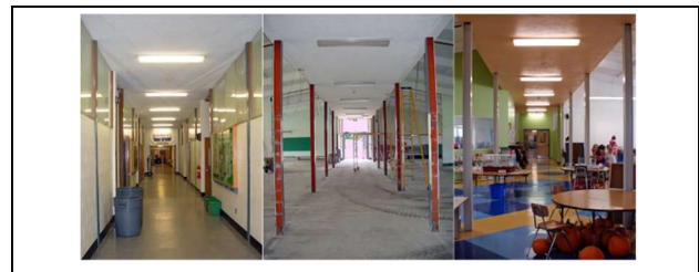
Figure 11: Renovation of double loaded corridor in Forest Avenue Elementary School wing [28].
