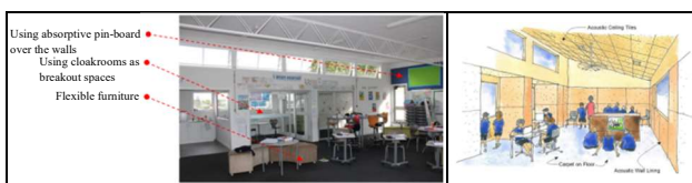
Figure 3: Interior perspective in renovated learning spaces of Avalon block and the most important indicators of internal acoustic treatments [19].
