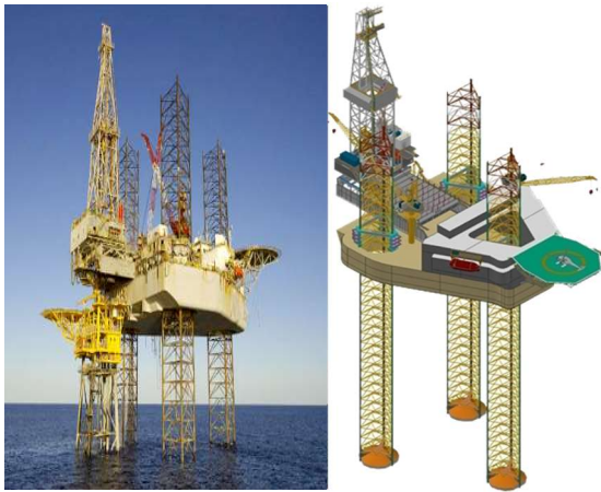
Figure 1: jack-up unit structure (Hambly, 1985) [10] [11].
