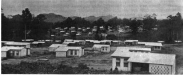
Photograph No. 4 Unfinished 'core houses' finished by guided self-help housing method in Ghana.
