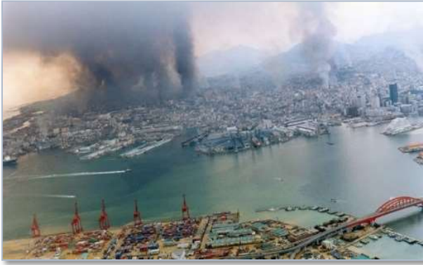
Figure 1: The Great Hanshin-Awaji Earthquake occurred in 1995 destroyed the old wooden buildings.
